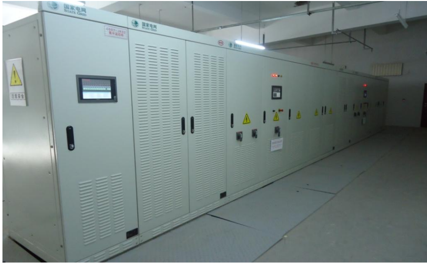
500kW PCS(Power Conversion System)
