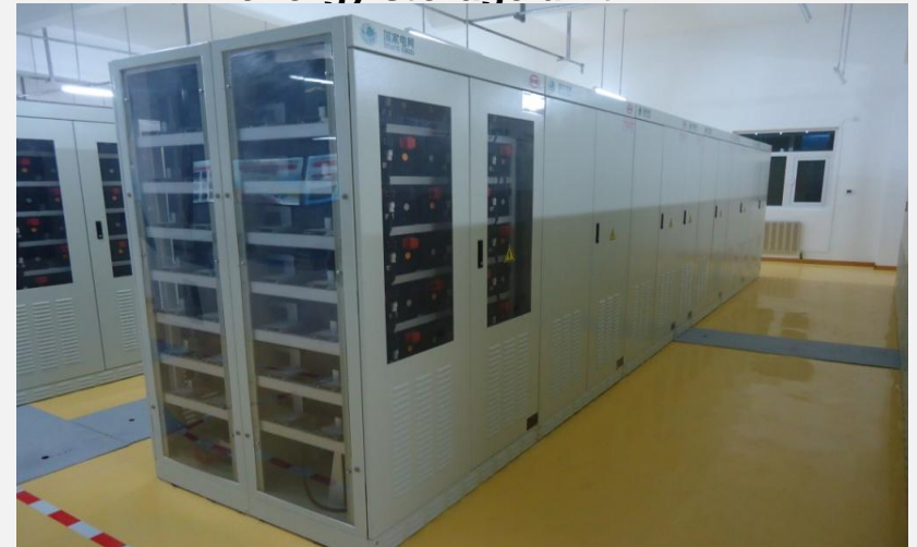
2MW energy storage unit
