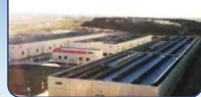
China State Grid 6MW ESS
